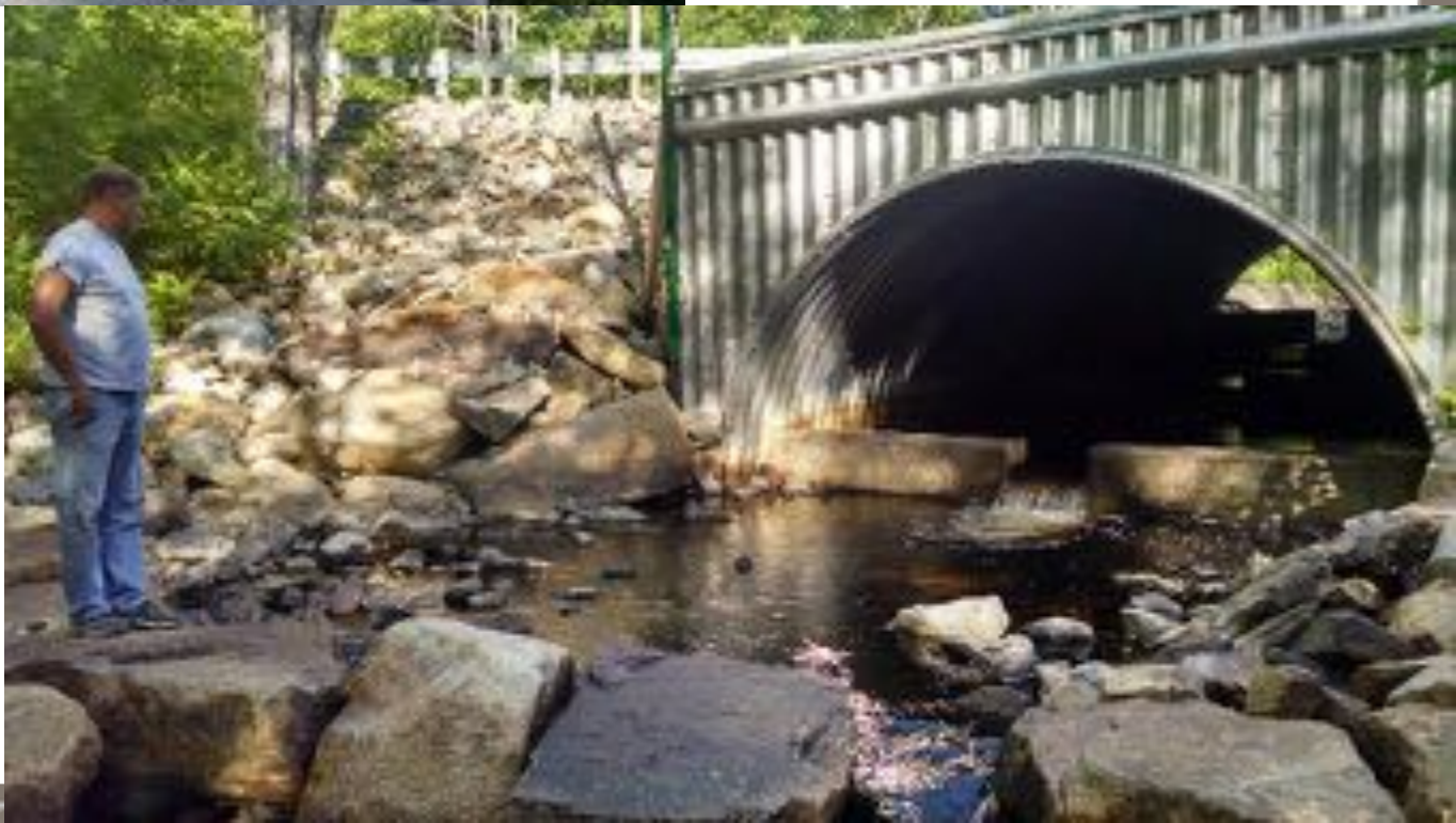
Flanders Stream Culvert Replacement
