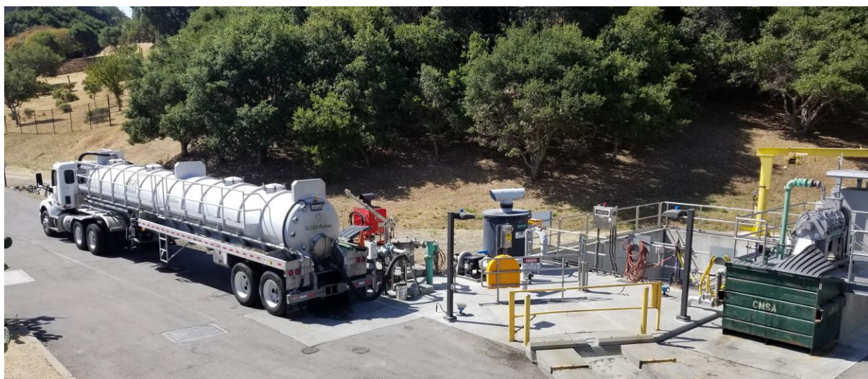
Figure 3. Truck offloading FOG at CMSA Organic Waste Receiving Facility. Source: CMSA.
