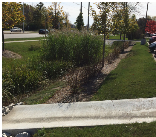
An example of a Bioswale
