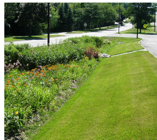
An example of a Bioswale
