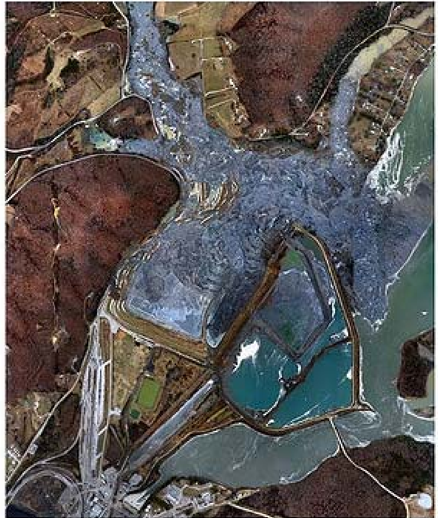
Aerial Image Of Kingston Ash Slide 12/23/08
