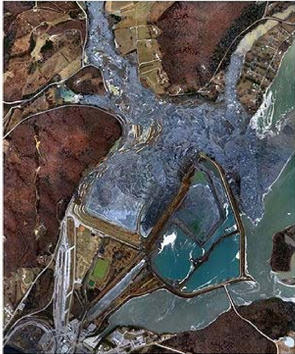
Aerial Image Of Kingston Ash Slide 12/23/08
