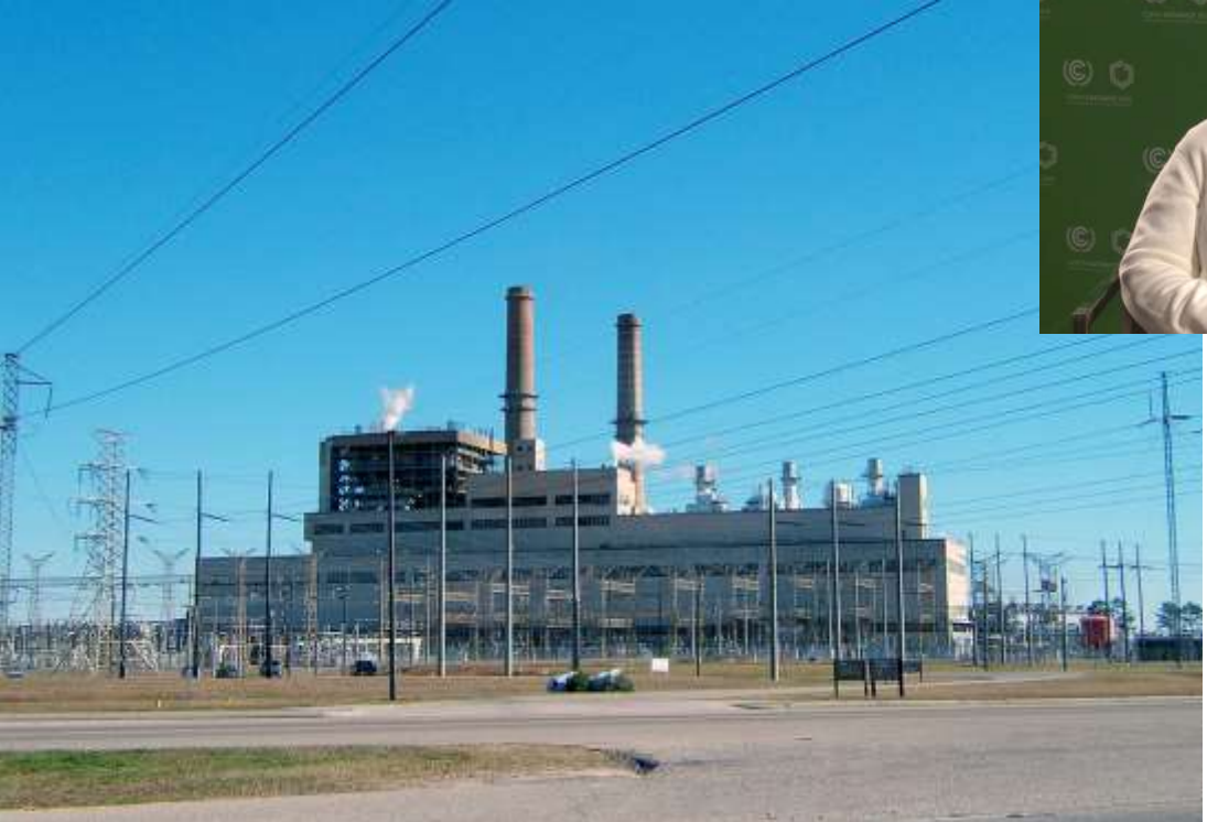
Jack Watson Electric Generating Plant
