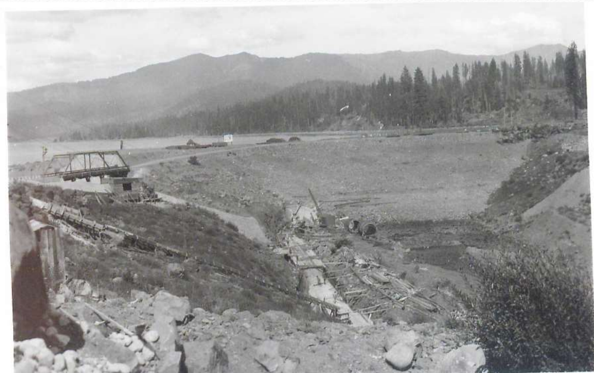
Big Meadows dam construction 1925 (Huber, WRCA)
