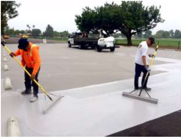
Two Coats of Guard Top Cool Seal are applied
