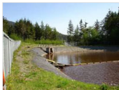
Figure 1. Landfill settling pond.
