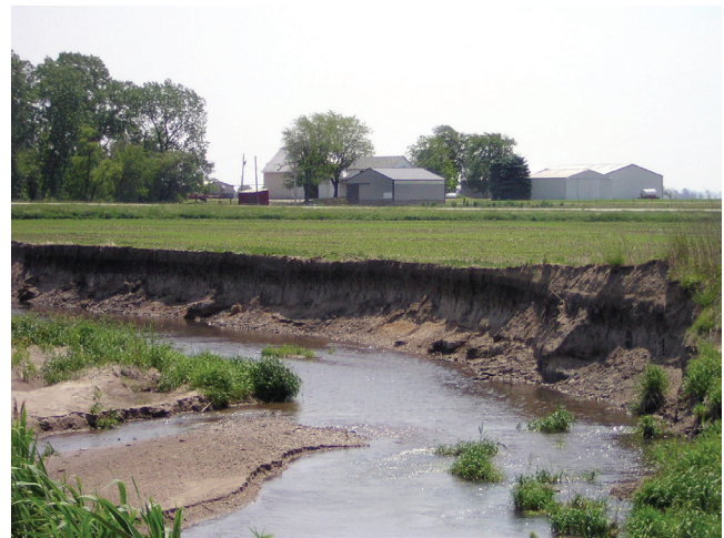
Figure 4.2. Lack of a riparian buffer and row cropping to the stream edge have led to stream bank failure and massive erosion along this stream in northwestern Indiana. Buffers of riparian vegetation stabilize stream banks and decrease sediment inputs to streams. (Photo courtesy of Todd Royer.)
