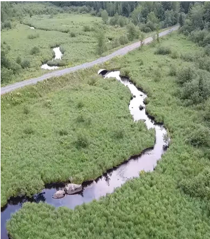
Aerial photo of the abandoned rail bed post-restoration. Photo courtesy of Mike Jones, Stockbridge-Munsee Community.
