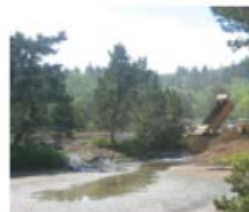
Figure 46. Filling interior ponds.
