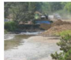
Figure 47. Filling interior ponds.
