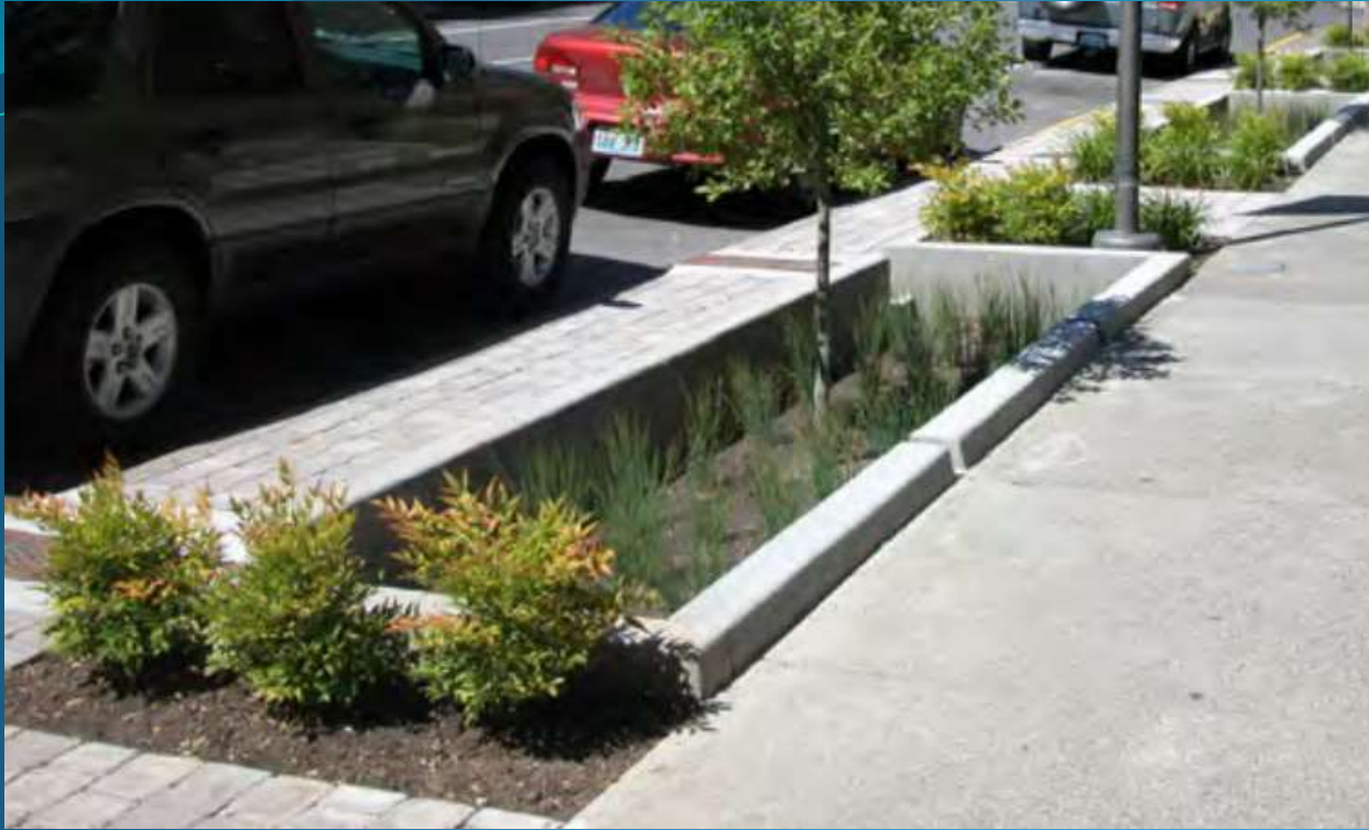
12 th & Montgomery Street, Portland, Oregon. Image Source: Low Impact Development Approaches Handbook by Clean Water Services, Portland Oregon.
