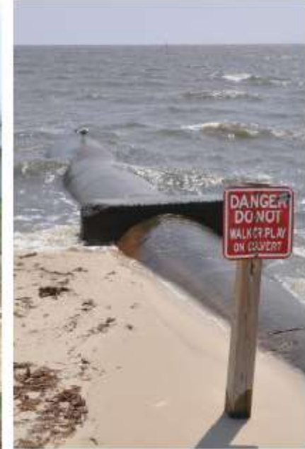
STORMWATER OUTFALL
